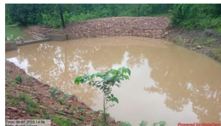
Water harvesting structure
